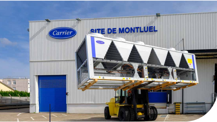
The Carrier site in Montluel
